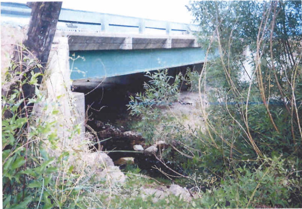
Culvert under US 36 at Coal Creek.
