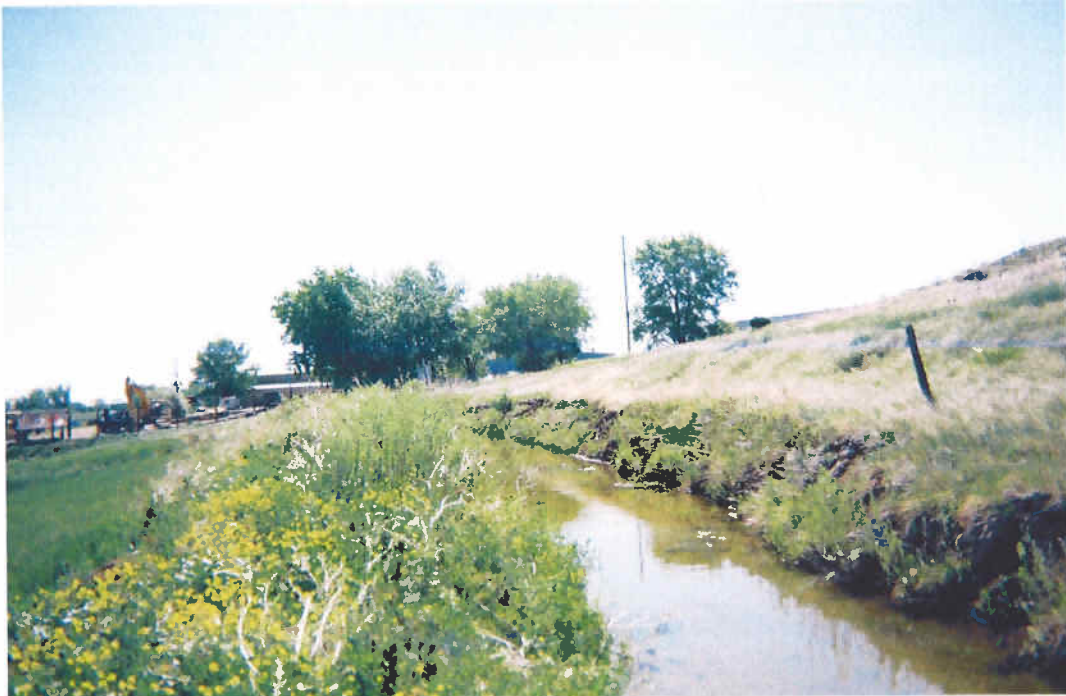
Enterprise Ditch where ditch parallels BNSF tracks (facing east).
