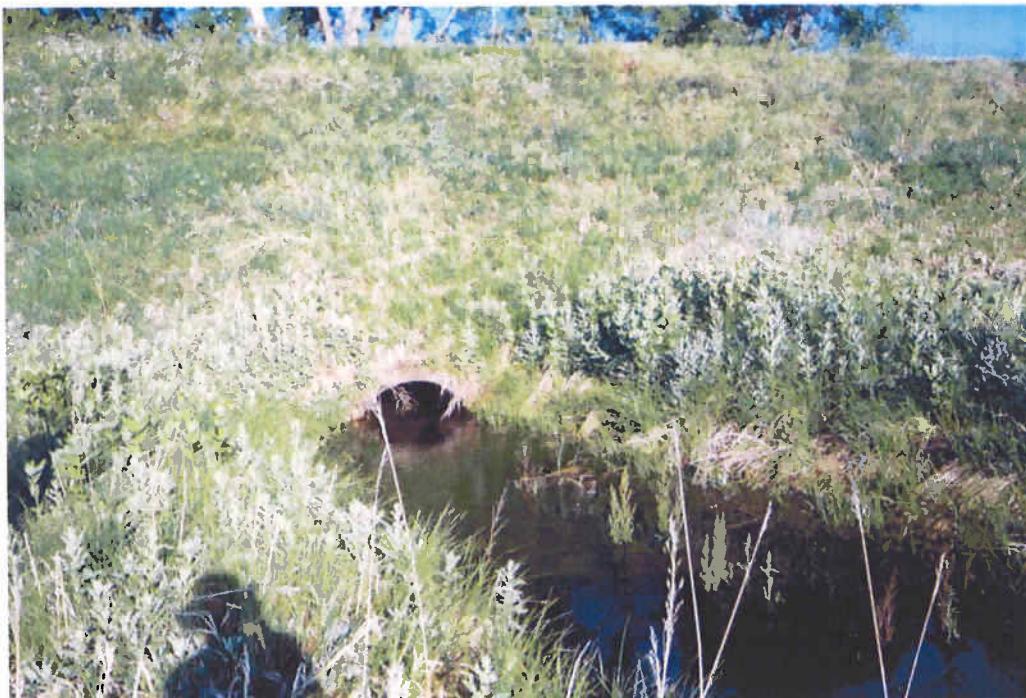
Pipe Culvert under Cherryvale Road on the North Side of US 36.
