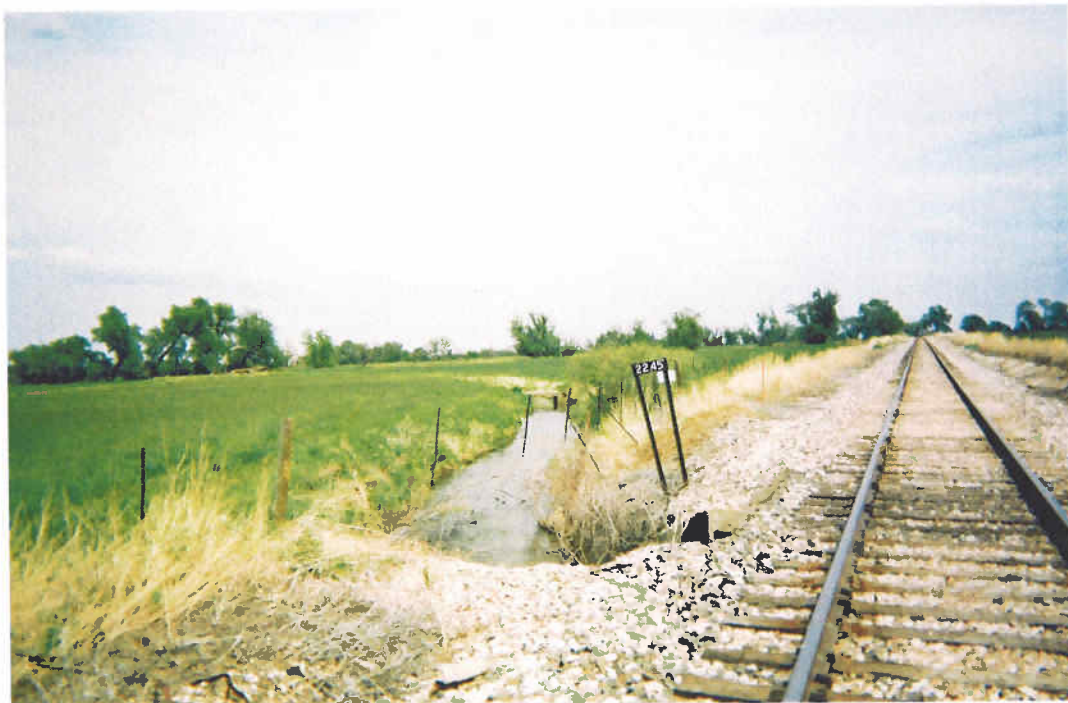
South Boulder Canyon Ditch at BSNF crossing (facing east).
