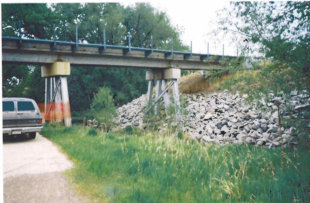
BNSF railroad bridge over Coal Creek (facing west northwest).
