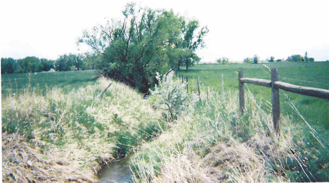
Marshallville Ditch on South Side of BNSF crossing (facing south).
