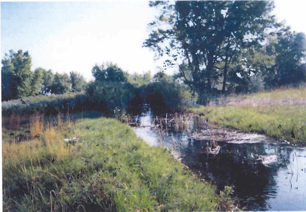
South Boulder Canyon Ditch on the Southwest side of US 36.
