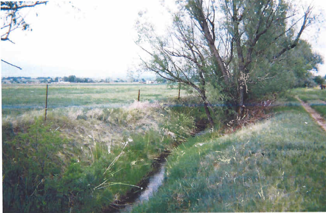
Marshallville Ditch on North Side of BNSF crossing (facing north)
