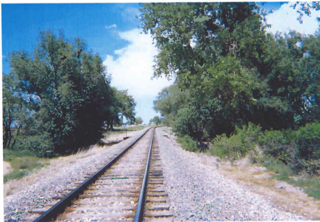
Fourmile Canyon Creek at BNSF Railroad Tracks (facing northeast).
