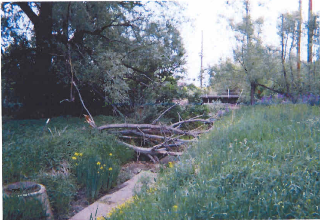
View of BNSF Railroad Bridge over Boulder Creek (facing north).
