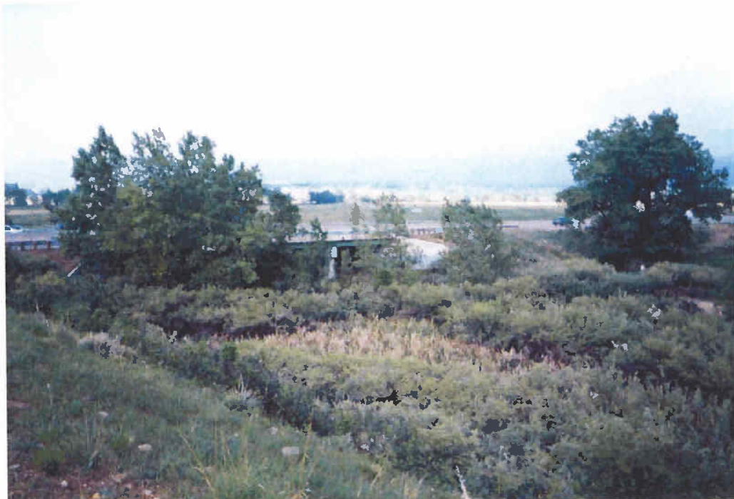
South Boulder Canyon Ditch (facing southwest toward US 36).
