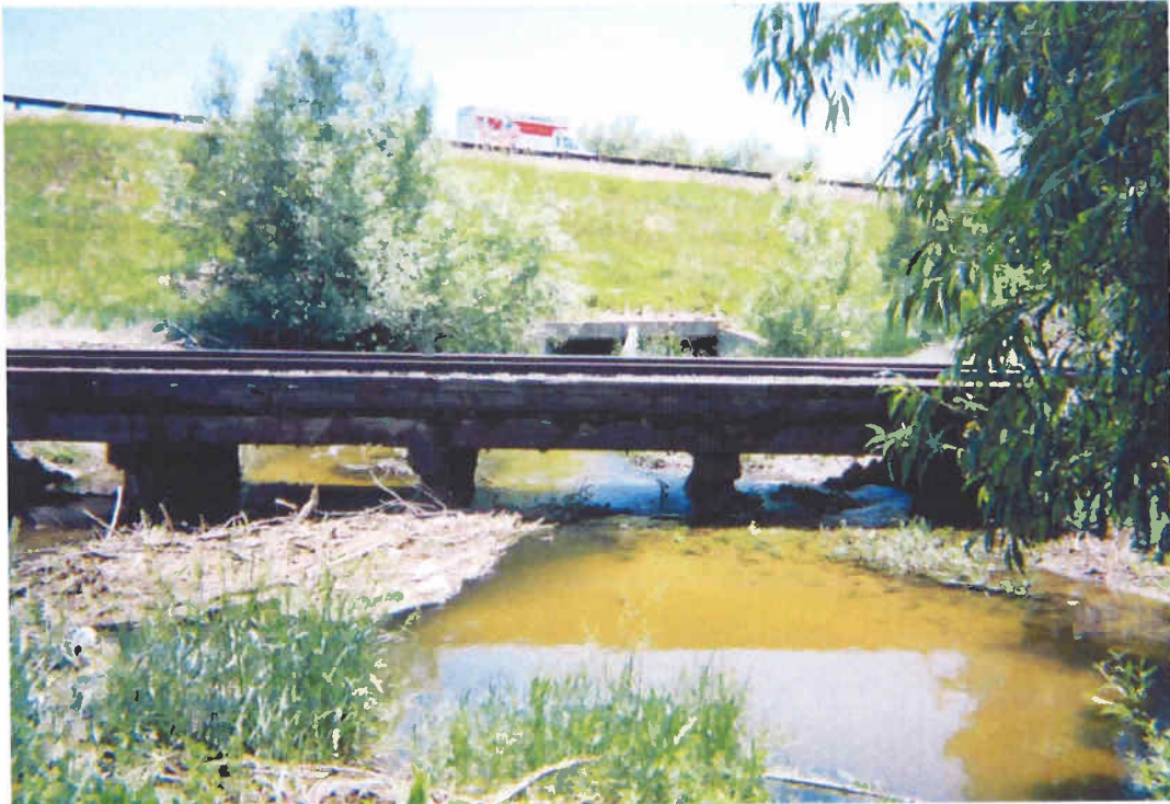
South Crossing of BNSF Railroad Tracks over Wonderland Creek (facing east).
