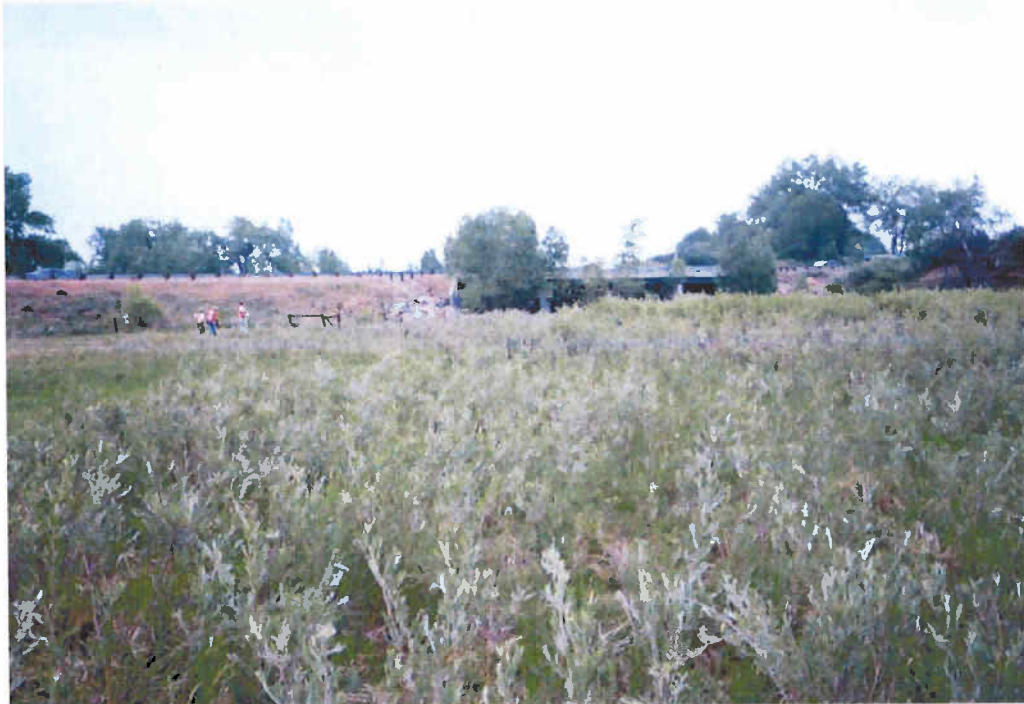
Bridge over South Boulder Creek (facing east)
