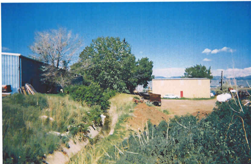
Enterprise Ditch, south of BNSF tracks (facing west)
