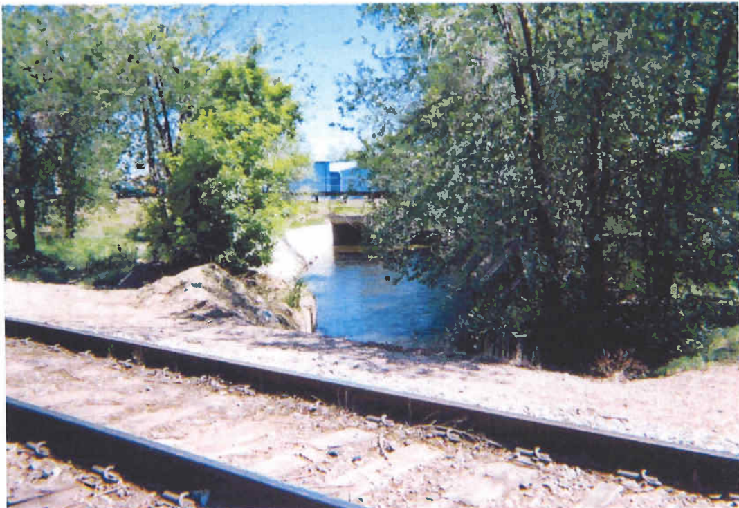
Boulder and Lefthand Ditch from BNSF Railroad tracks (facing east).
