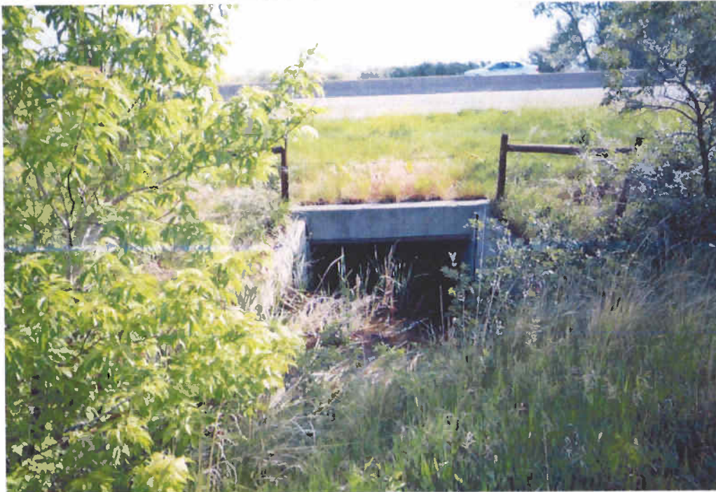
Culvert under Marshallville Ditch on southwest side of US 36.
