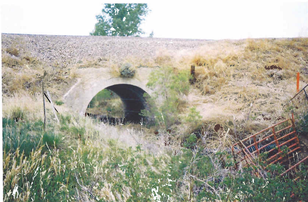
Rock Creek Culvert under BNSF tracks (facing west).
