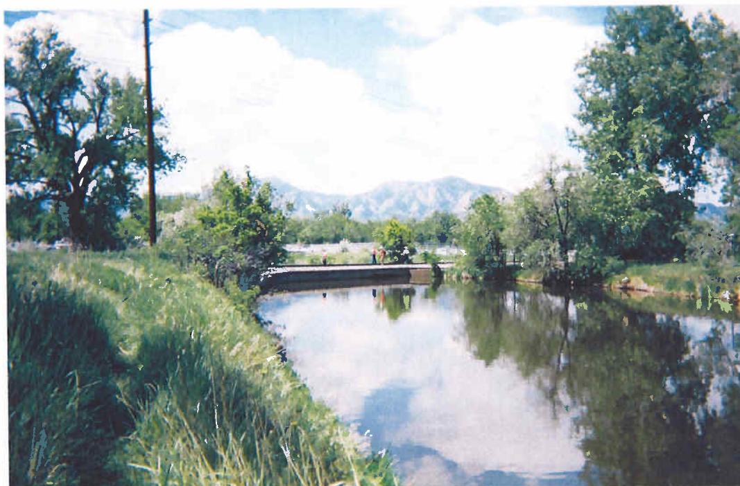
South Boulder Creek Inlet Canal to Leggett Reservoir (facing north from bridge)
