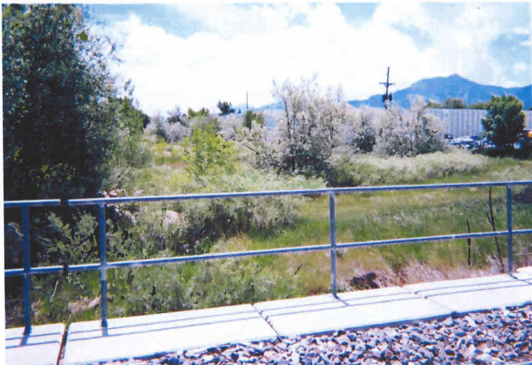
BNSF Bridge Crossing over Dry Creek No. 2 Ditch (facing north).
