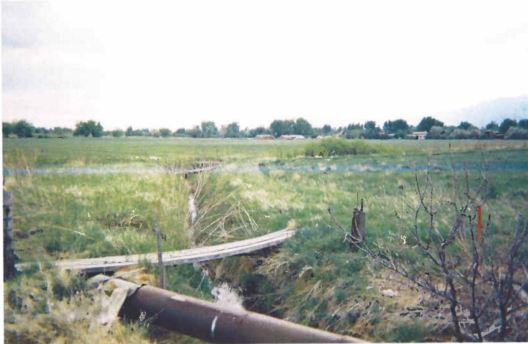
City of Boulder Burke-Hodgson Lateral at BNSF crossing (facing west-southwest).
