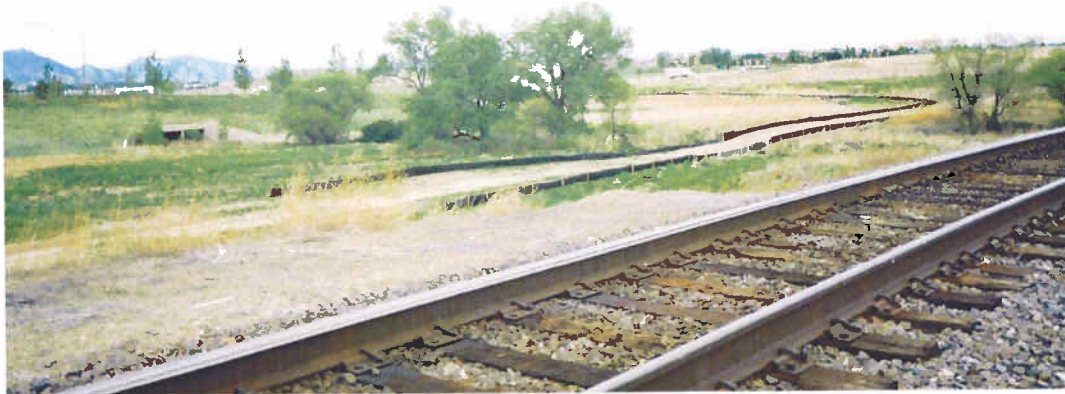
BNSF tracks at Rock Creek (facing northwest).
