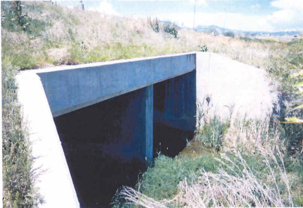
View of Rock Creek Culvert under North Side of US 36.
